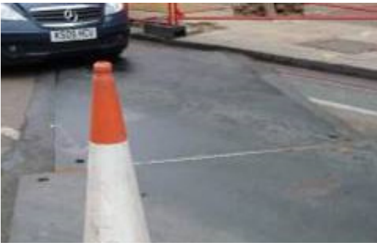
Figure 12 - Innovative use of welded steel plates
