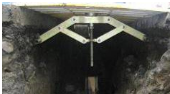
Figure 9 - Road plate fixing and support system
